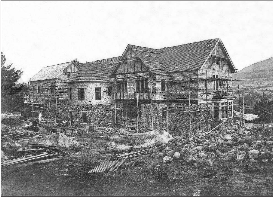
Wellscroft under construction, 1903.
