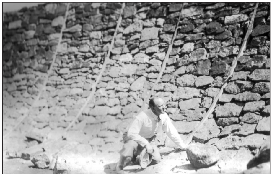
In September 1930 an Olympic official examines the high stonework on Shady Corner, one of the three hairpin curves on the 1932 Olympic bobsled run on Mount Van Hoevenberg.
