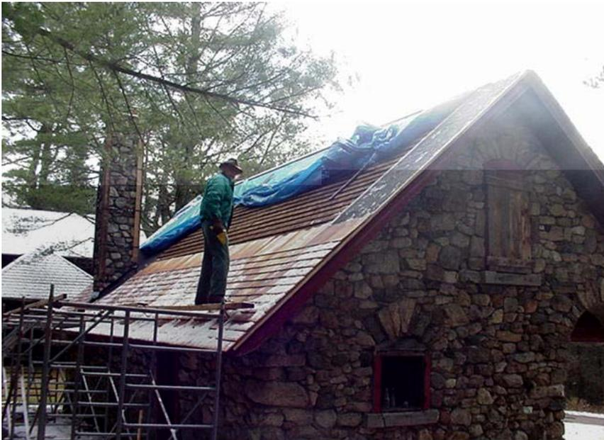
*Late in the fall of 2001, the Department of Environmental Conservation crew resumed work at the Santanoni farm. A new red cedar shingle roof was installed on the Creamery and the deteriorated wing on the Main Barn was stabilized and reroofed. Clive Friend is shown here working on the Creamery.
